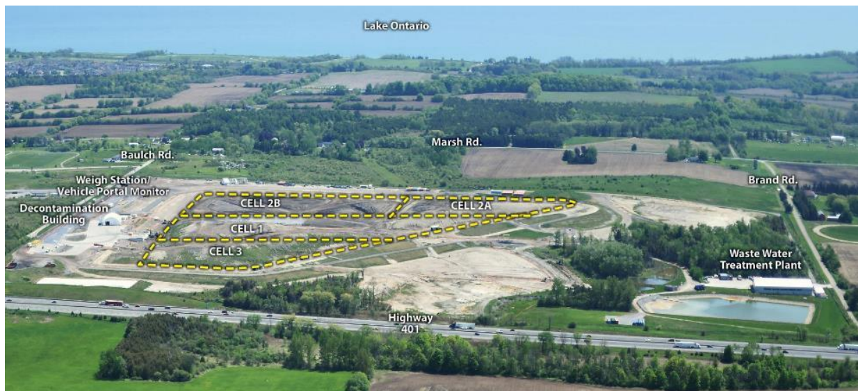
Figure 2: Port Hope Project Long-Term Waste Management Facility
