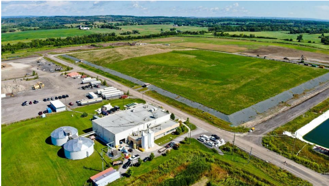
Figure 1: Port Granby Engineered Containment System and Waste Water Treatment Plant
